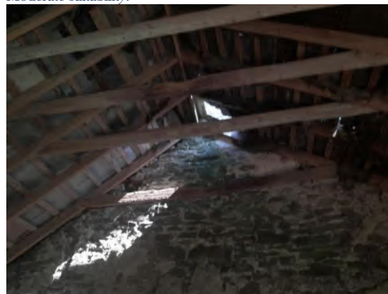
Plate 4-24 Felt underlining and damaged roof offering access and roosting potential for bats.
